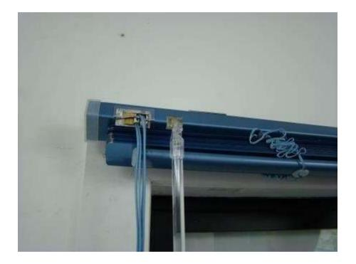
• This is how it should look once completed. Pull the cords toward the middle of the blind, this releases the cord lock allowing you to lower the blind. Use the wand to control the angle of the slats.
